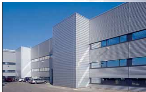
Two groups of Lean-Lifts® spanning multiple floors were docked onto the building from the outside so that production area wasn't sacrificed
